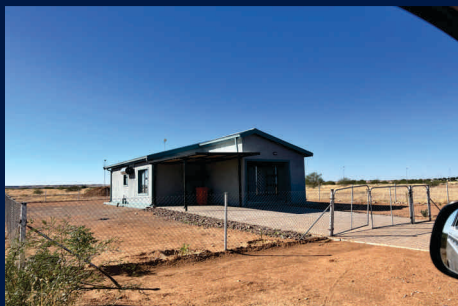
Mariental Extension 6 Housing Development
